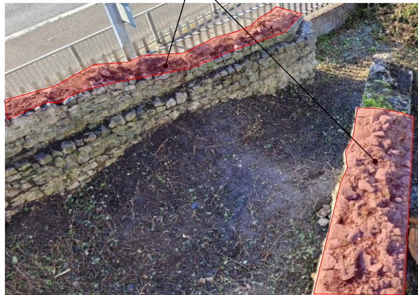
Area between Flanking Walls viewed from the top of the Arch
