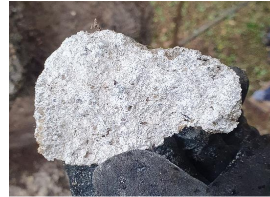
Existing lime-rich mortar on site
