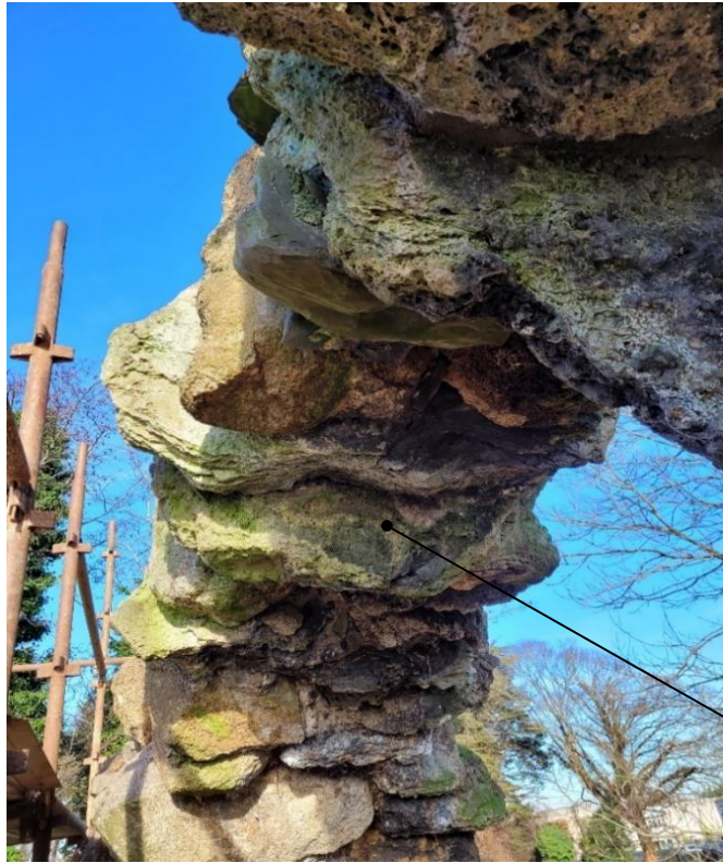
Underside of North-West side of Arch
