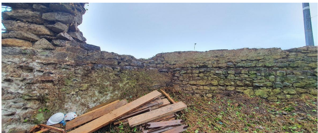
Figure 10 – Inner face of southeast flanking wall
