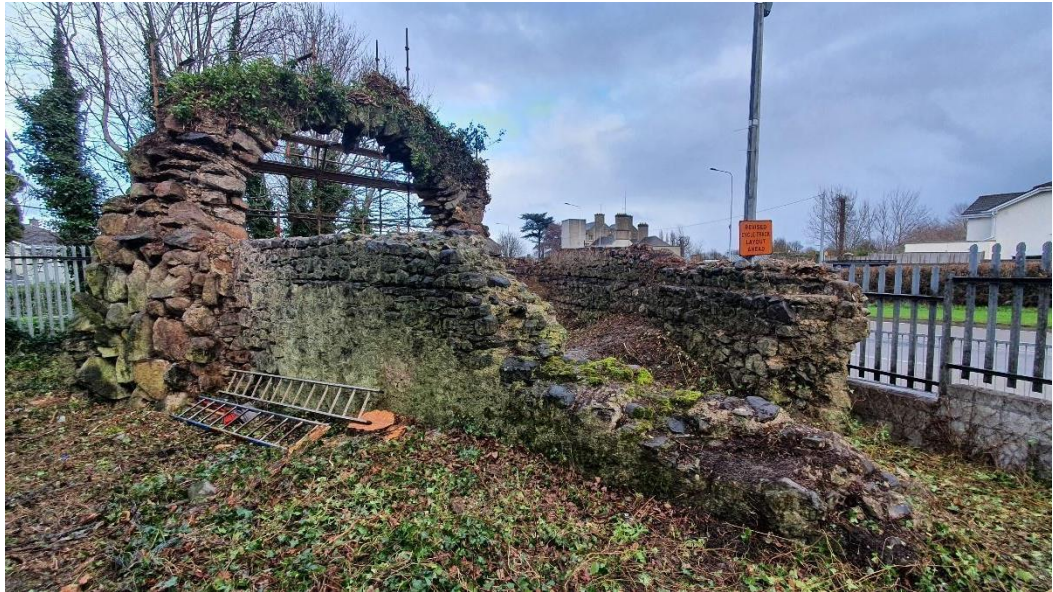
Figure 1 – Arch and flanking walls during vegetation removal
