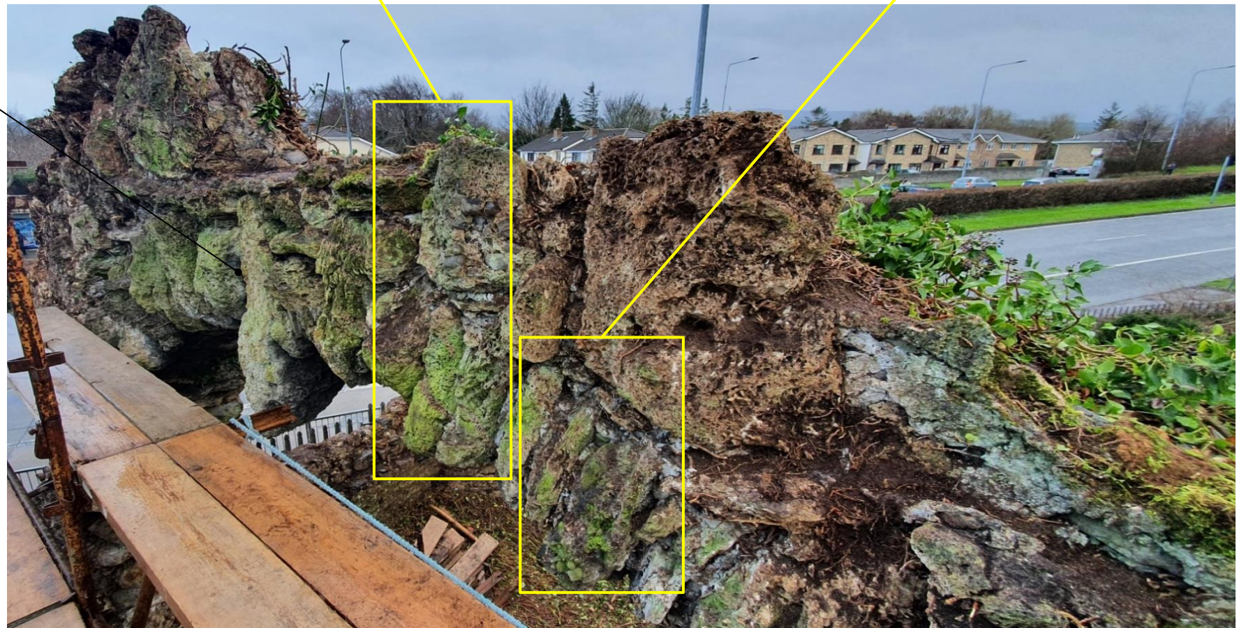
Top of North-East side of the Arch
