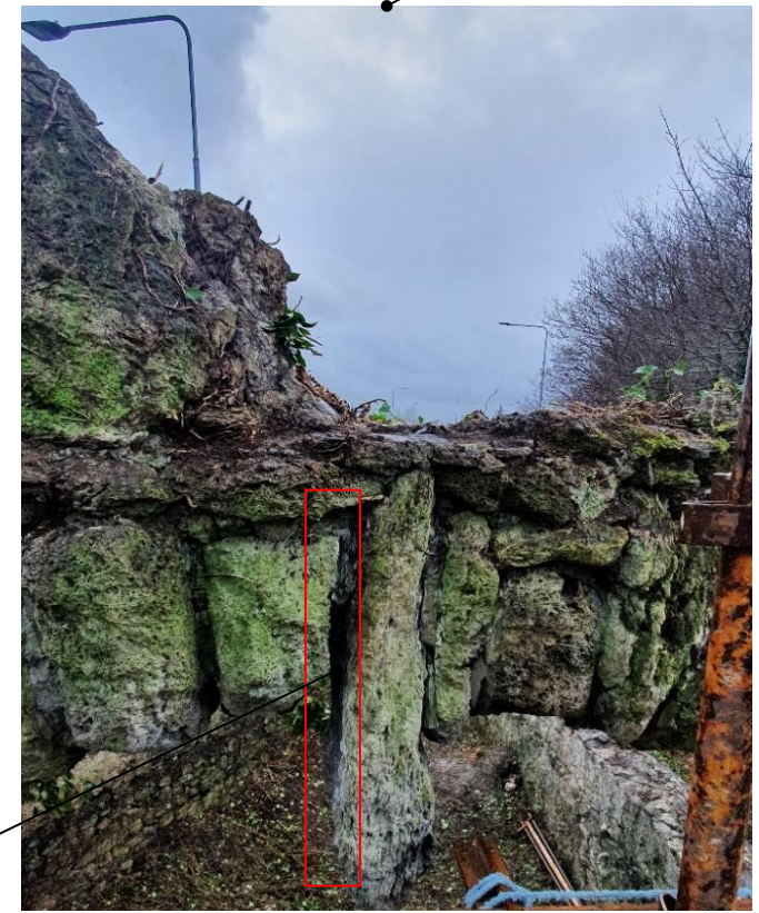
Image of missing stone on top of Arch
