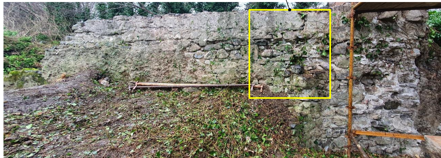
Inner face of North-West Flanking Wall
