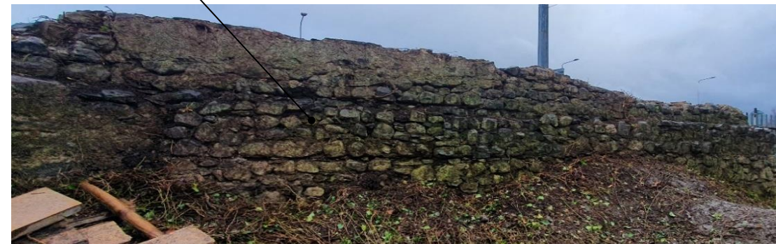
Inner face of South-East Flanking Wall
