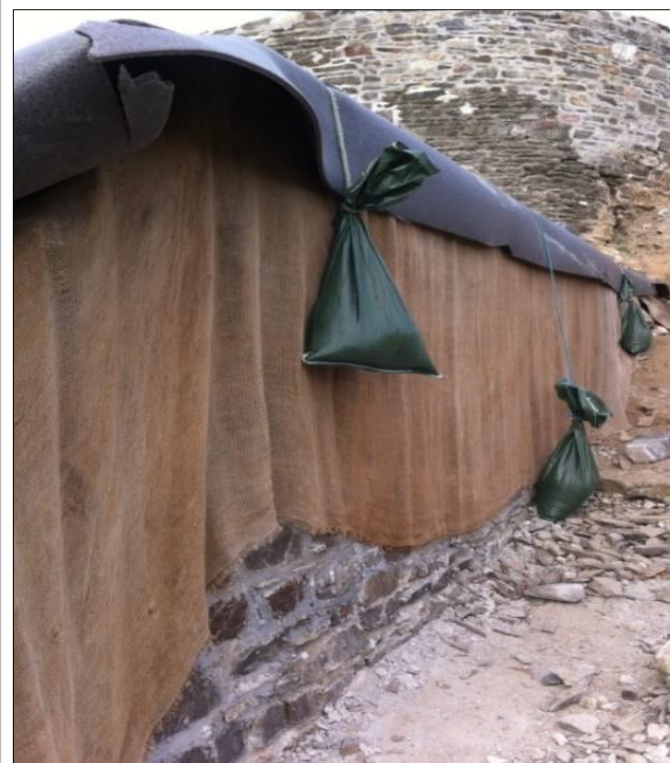
Example of appropriate protection to allow wall to dry out yet not become saturated by rain on upper surfaces
