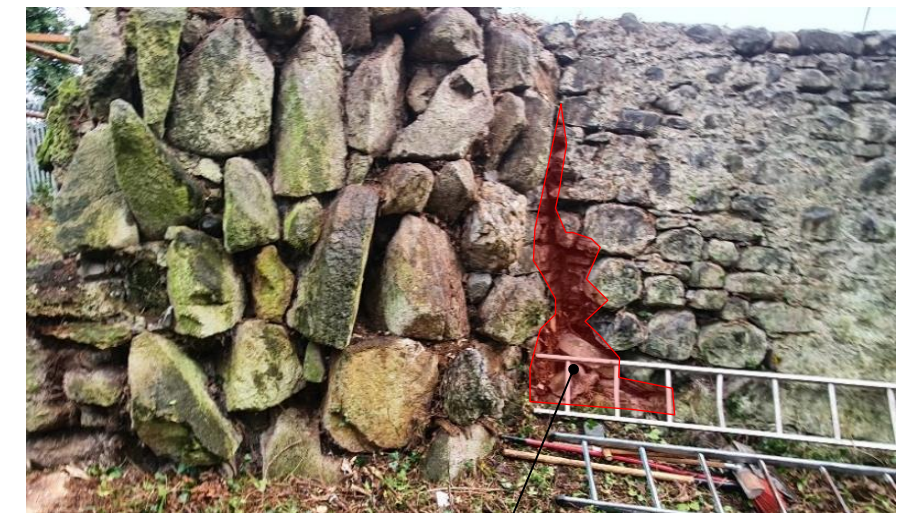
Outer face of North-West Flanking Wall
