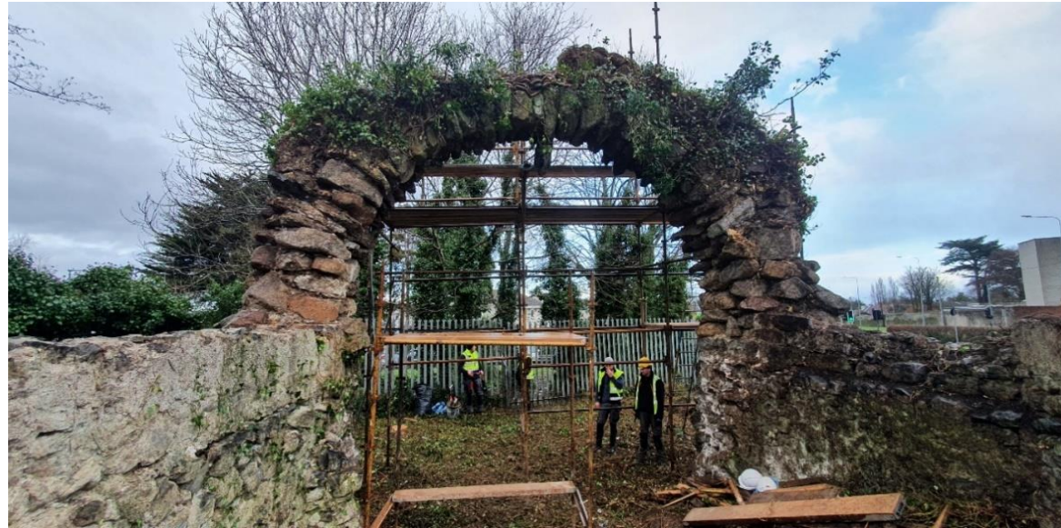
Arch during vegetation removal viewed from South-West
