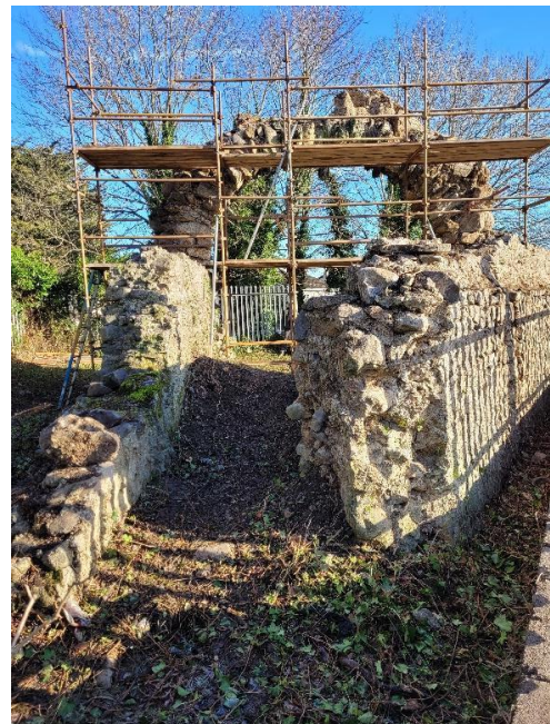
Figure 9 – Arch and flank walls after vegetation removal
