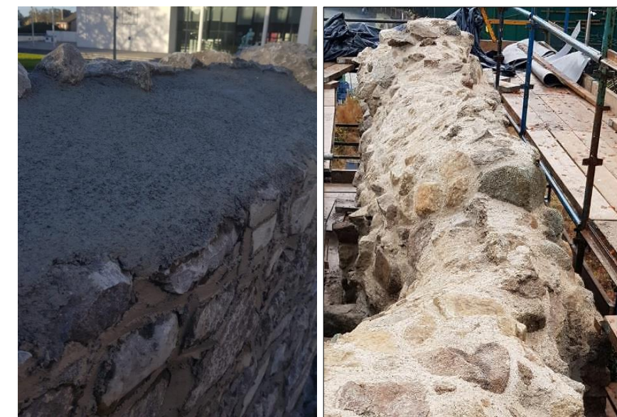
Sample of regularised (left) and rough-raked (right) wall top finish
