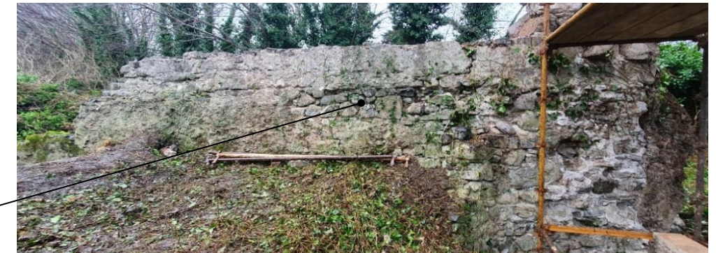
Inner face of North-West Flanking Wall
