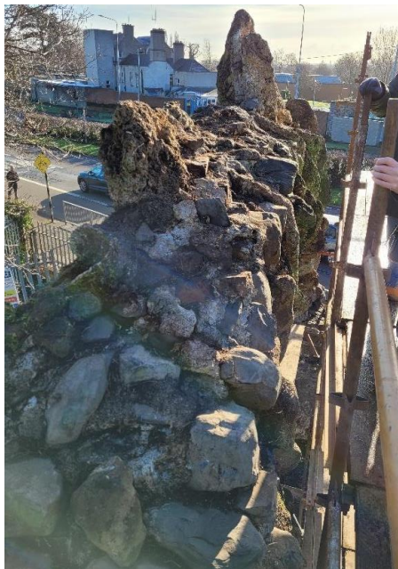
Figure 7 – Top of arch after vegetation removal
