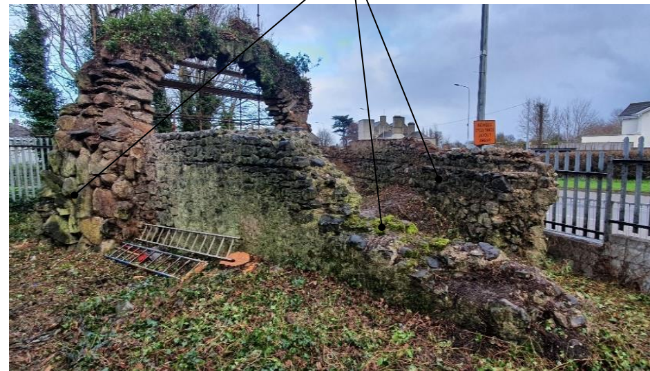
Arch and Flanking Walls viewed from North-West
